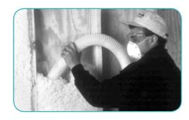
Benefits: InsulSafe SP is noncombustible, noncorrosive and odor free. In addition, InsulSafe SP won't settle, contains no chemicals to cause mildew and fungus growth, contains no formaldehyde, provides no sustenance for vermin, contains no asbestos, won't rot or decay and won't absorb moisture. Insulsafe SP improves energy efficiency and reduces energy consumption. This product helps conserve nonrenewable energy sources, reduces dependence on foreign oil and reduces greenhouse gas emissions.
